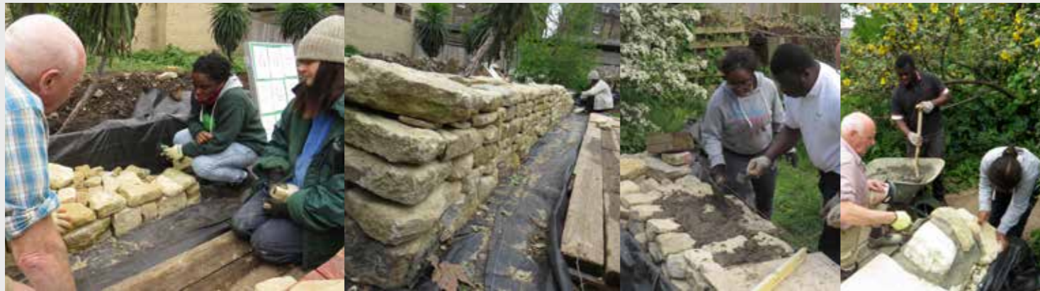
Careful planning and consideration is needed when choosing and placing stone. The wall nears completion, though it needs capping: slabs donated from Chelsea Flower Show are cemented in place as seating. The final wall with workers, Susana, Serafina, Joel.
